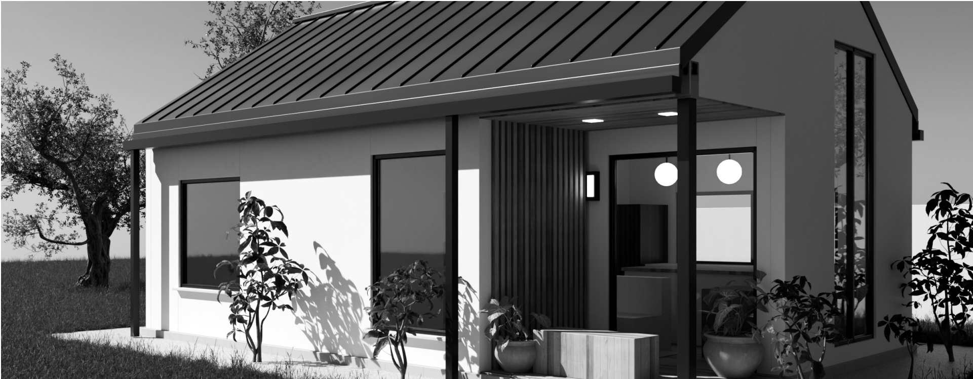
A Porch corner The 8' x 6' porch is cut out of the volume, so the roof and gable carry over it on a single steel post.
